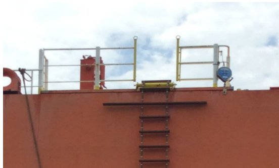
Figure 2: Gap in handholds appear to accommodate spreader.
