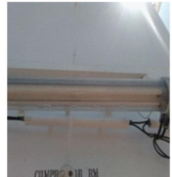
*Standing Water in a Certified Safe Flameproof Light Enclosure Indicating Failed Ingress Protection*
