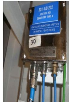
*Improper Cable Gland Installation/Modification*
