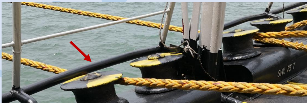
Figure 2: Arrow showing the bent railing above the roller fairleads at the aft mooring station
